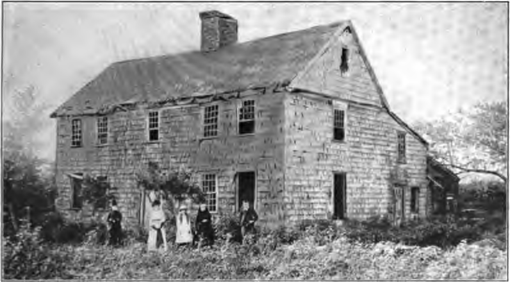
MOSES WHEELER HOMESTEAD. BUILT BEFORE 1700
