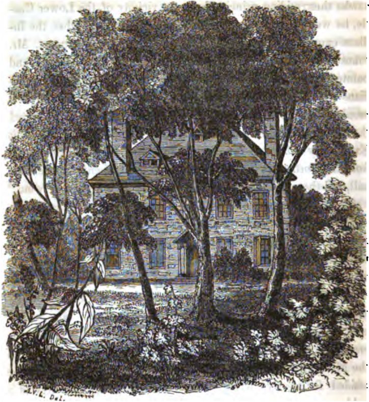
SOUTH VIEW OF FORT JOHNSON.
