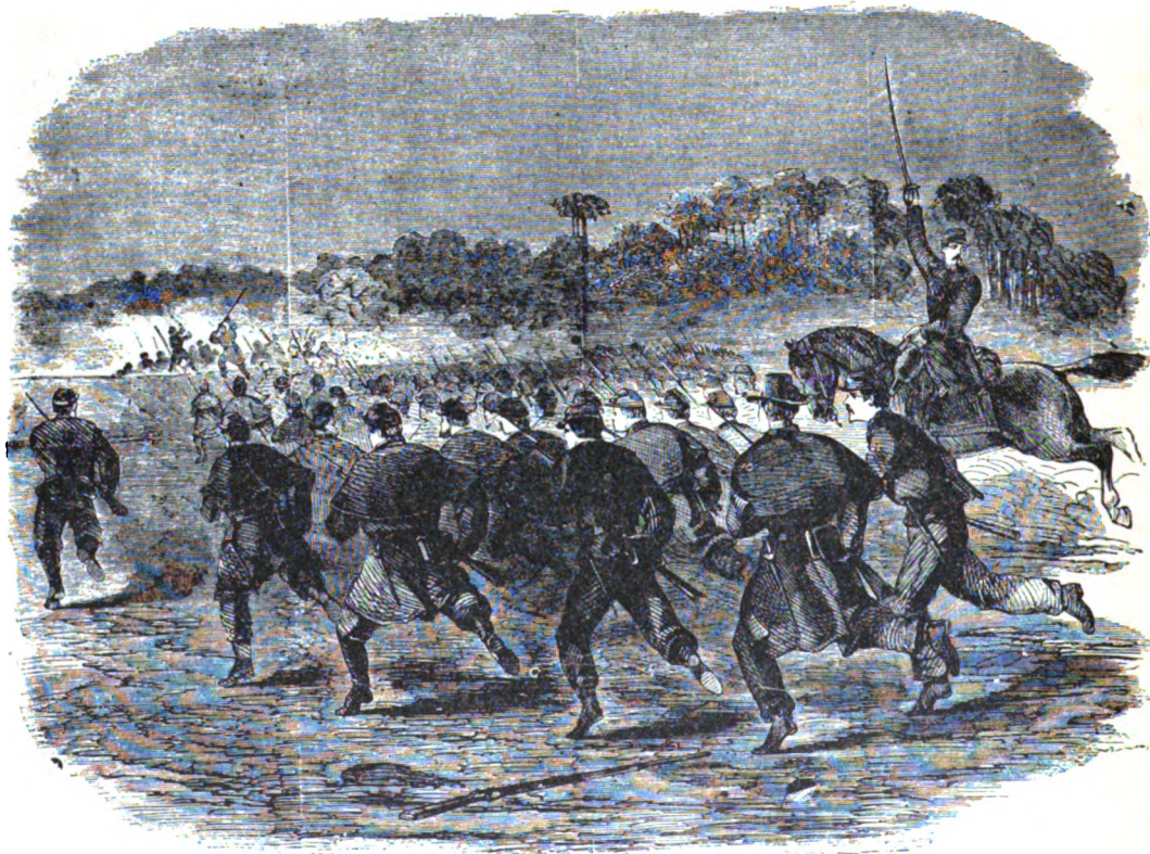
THE 1ST MASSACHUSETTS AT WILLIAMSBURG
