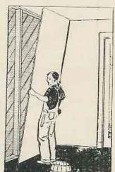
Sheetrock, the fireproof wallboard, is standardized building material—uniformly \(^3\)/s-inch thick—standard widths—standard ceiling-high lengths. Nails right to joists and studs, or over old walls and ceilings.
